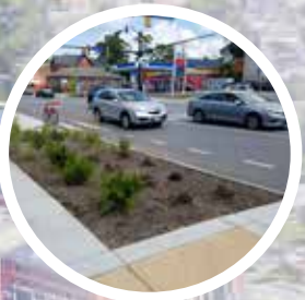
Rain gardens along Niagara Street absorb and capture stormwater runoff.
