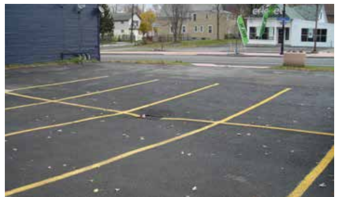
Two porous parking lots were created on City-owned vacant parcels as part of a Fillmore Avenue streetscape project.
