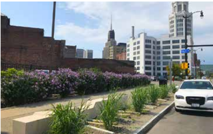
Rain gardens installed along Genesee Street helped transform the major corridor into a welcoming gateway from the city's East Side to downtown Buffalo.
