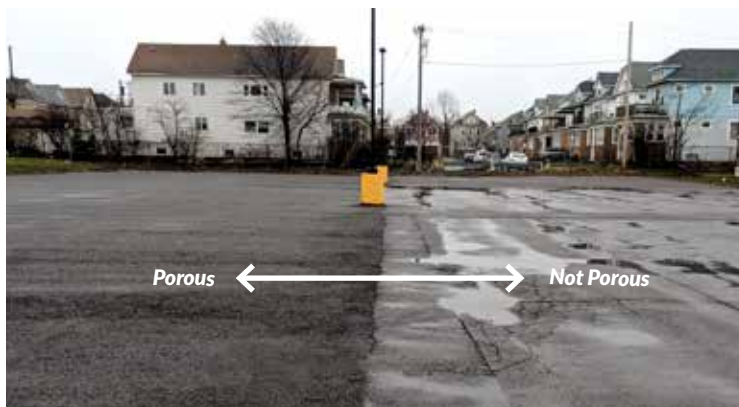
During a rain or snowmelt event, porous pavement in the expanded parking area at North Buffalo Ice Rink absorbs water beneath the ground (on the left side of the image), while water puddles on the ground in the older asphalt parking area (on the right).
