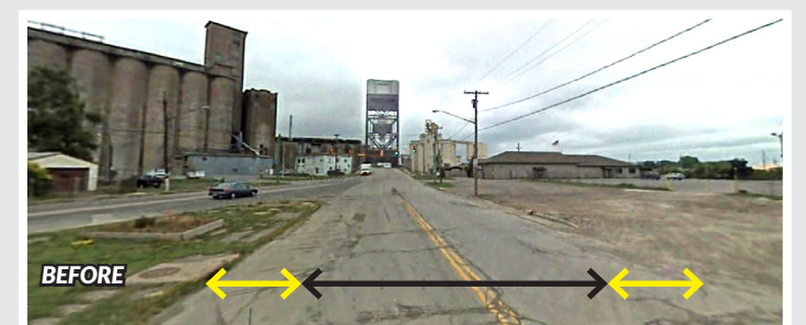
Road diet measures on Ohio Street reduced over 3.2 acres of impervious surface and allowed for a shared-use path to be built for pedestrians and bicyclists.
