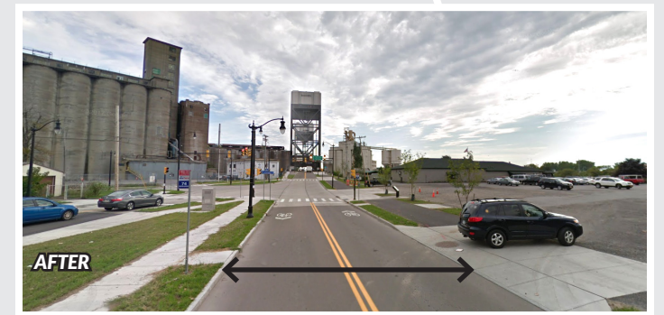
Road diet measures on Ohio Street reduced over 3.2 acres of impervious surface and allowed for a shared-use path to be built for pedestrians and bicyclists.
