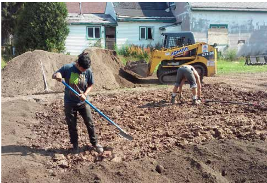
Figure 3.2: Green post-demolition for enhanced stormwater performance
