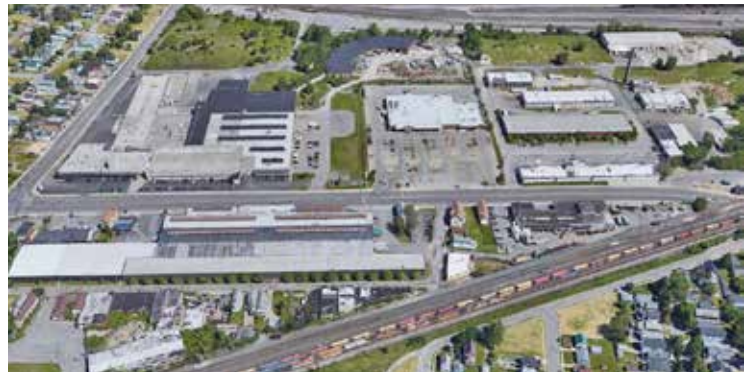
Figure 33.8: CSO Basin 33 has a number of large corridors that are flanked by larger commercial or industrial land uses and example is seen here at the intersection of Bailey Ave and Broadway
