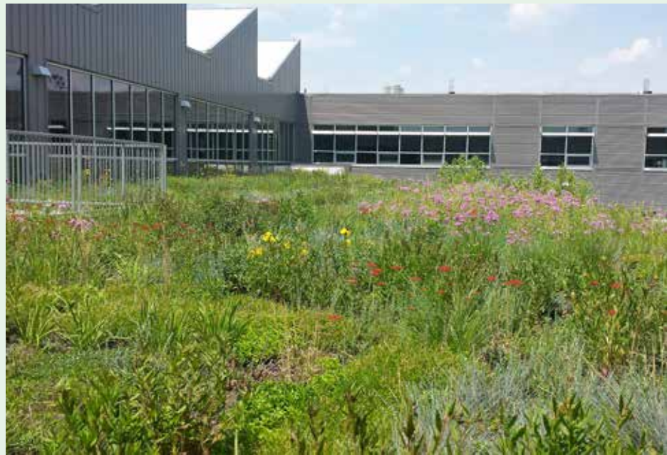
Figure 2.6: Green roof at Kensington High School in Philadelphia, PA (image ROOFMEADOW).
