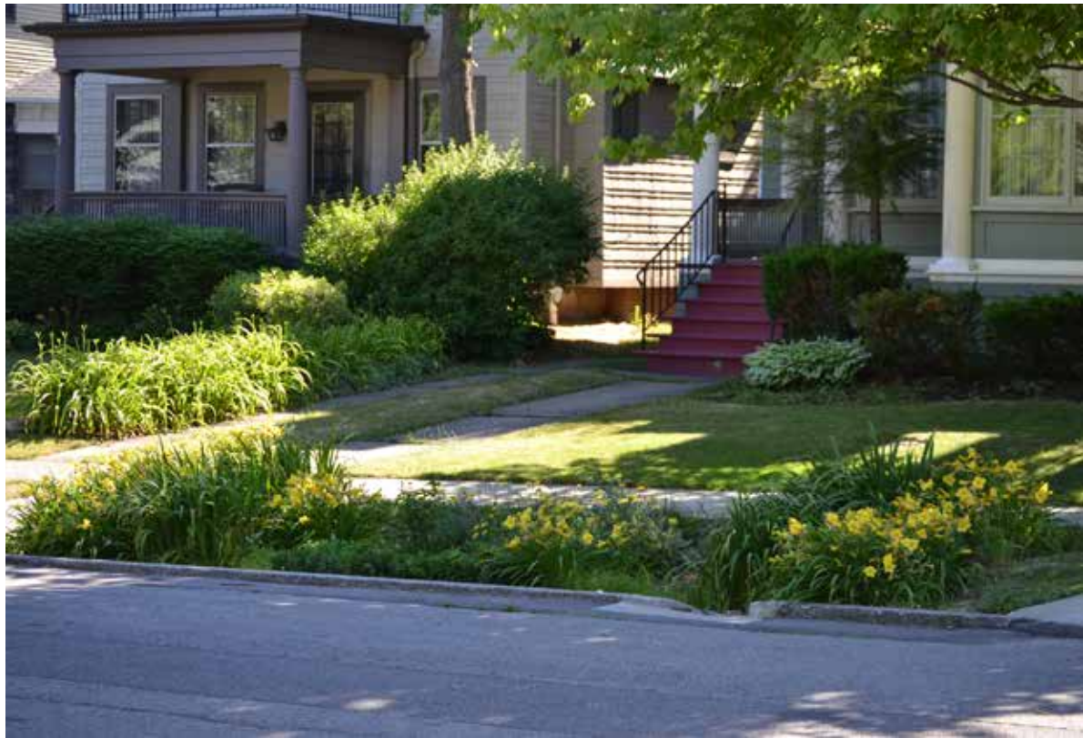
Figure 2.5: Buffalo Sewer Rain Garden on Windsor Avenue.
