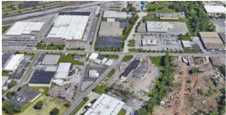
Figure 27.7: The north end of CSO Basin 27 is characterized by large commercial and industrial sites flanking William Street with large flat roofed buildings and big parking lots.
