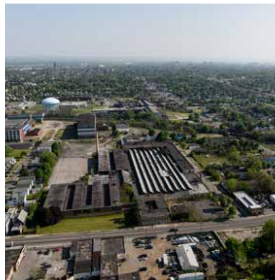
Figure 53.4: BUDC Redevelopment prior to demolition.
