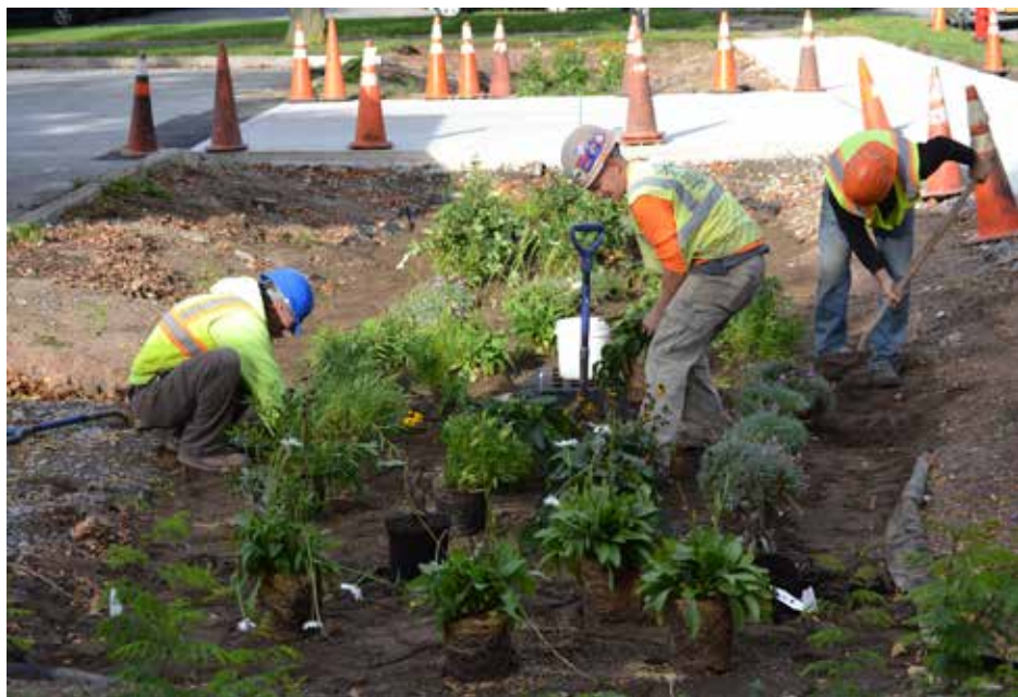
Figure 3.12: Workers installing a rain garden facility at JFK community center.
