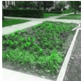
Figure 2.9: Rain garden along Windsor Avenue.
