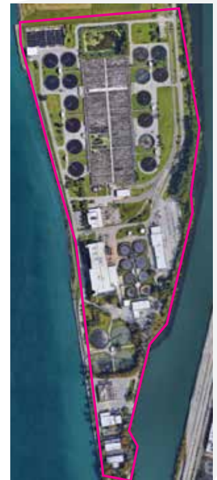
Figure 2.1: Buffalo's Wastewater Treatment Plant on Bird Island.
