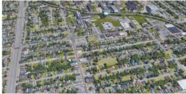
Figure 53.6: Kensington Expressway and a CSX rail line are examples of how infrastructure isolates neighborhoods and reduces walkability
