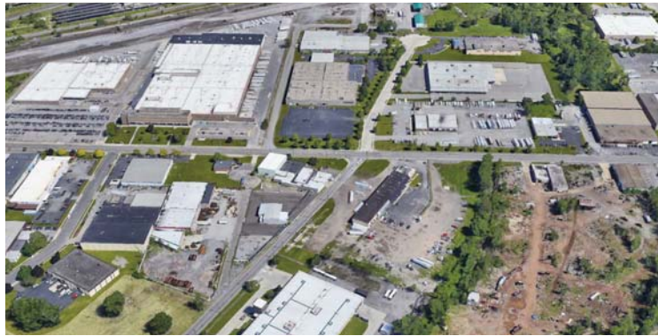
Figure 27.7: The north end of CSO Basin 27 is characterized by large commercial and industrial sites flanking William Street with large flat roofed buildings and big parking lots.
