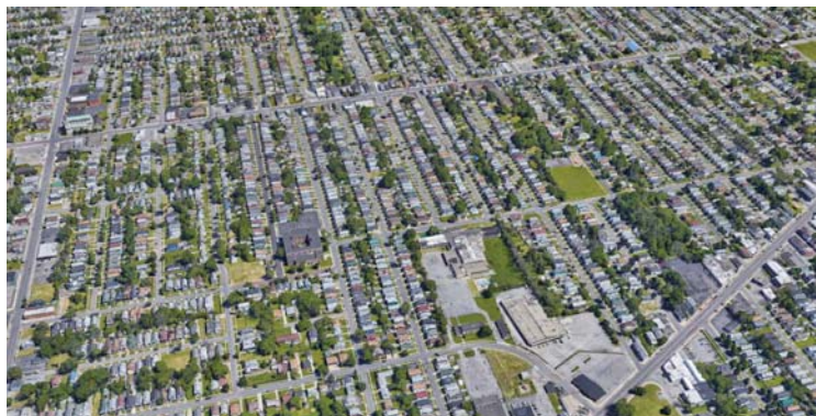
Figure 53.8: Dense single family detached housing comprises large pockets of CSO Basin 53 seen here in the eastern neighborhood of Kenfield.
