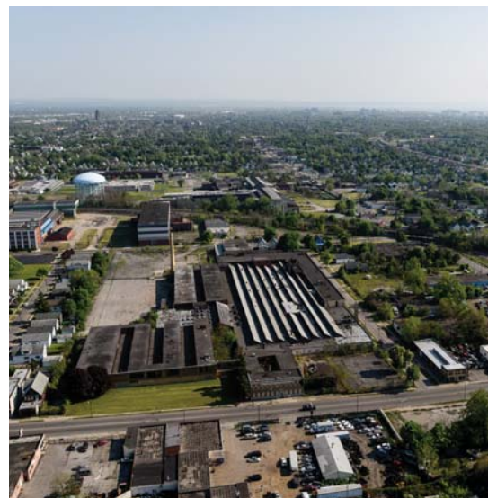
Figure 53.4: BUDC Redevelopment prior to demolition.
