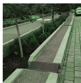
Figure 2.10: Porous paving alongside a bioswale.
