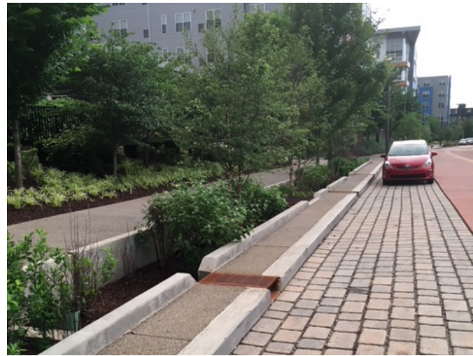
Figure 2.7: Porous paving next to bioswale along Living Place in Pittsburgh PA.
