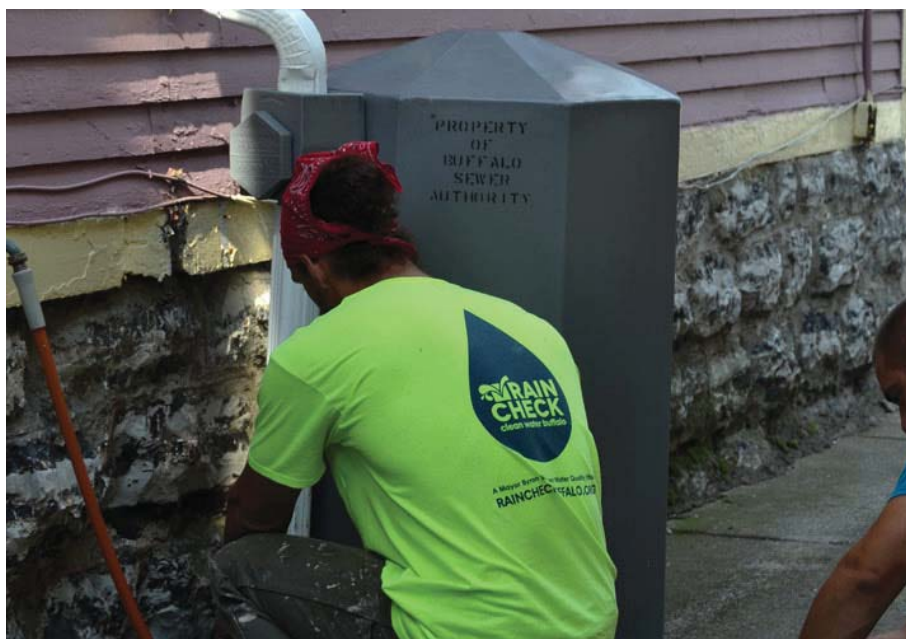
Figure 3.15: Rain Check rain barrel being installed at a residential property..
