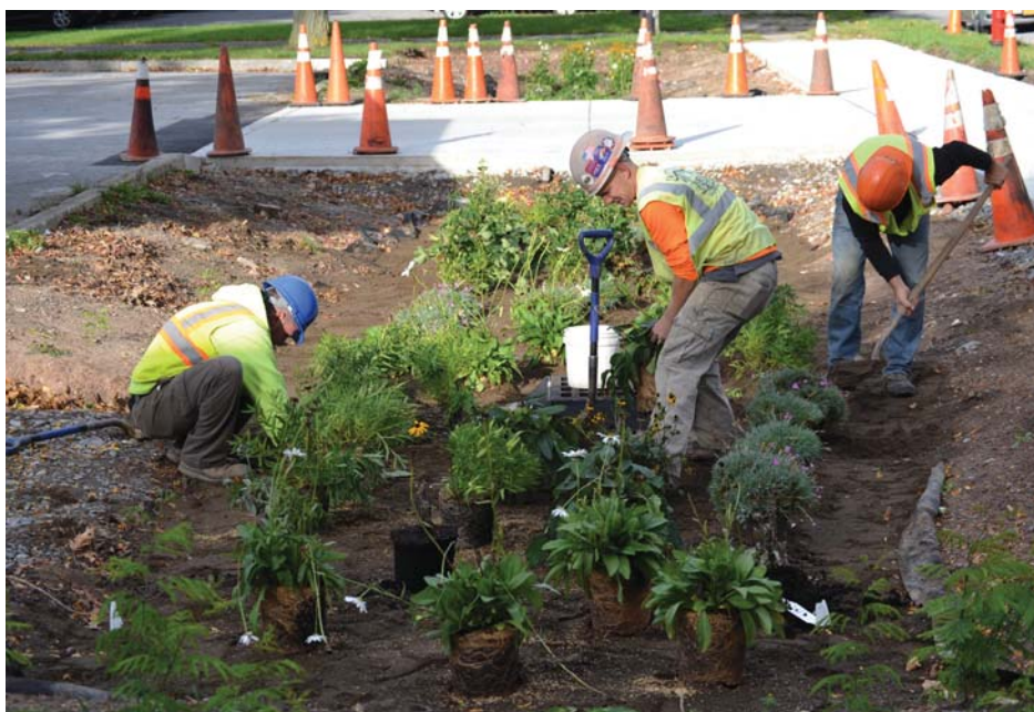
Figure 3.12: Workers installing a rain garden facility at JFK community center.
