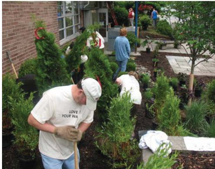
Figure 3.16: Team installing green infrastructure at the Crane Library.
