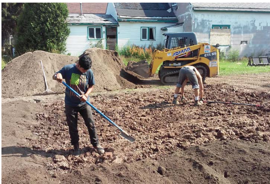
Figure 3.2: Green post-demolition for enhanced stormwater performance
