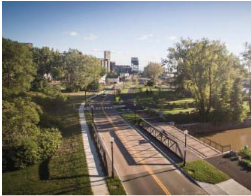
Figure 3.3: Green Street Case Study at Ohio Street.
