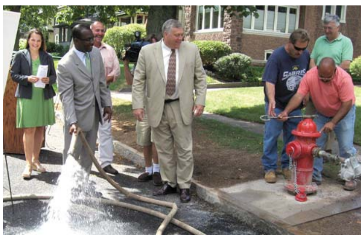
Figure 3.14: Demonstrating porous asphalt on Clarendon.
