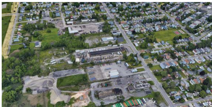
Figure 28.9: Along Hopkins and Abby street light industry borders the residential community and creates a barrier to open space to the west.
