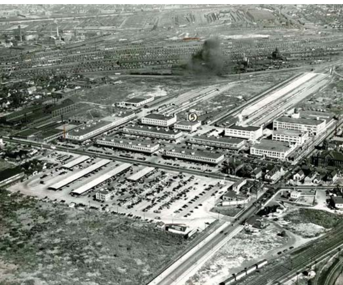
Figure 33.3: Historic image of Buffalo Food Terminal
